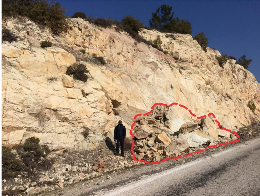
Figure 3. Planar failure observed in the field.
